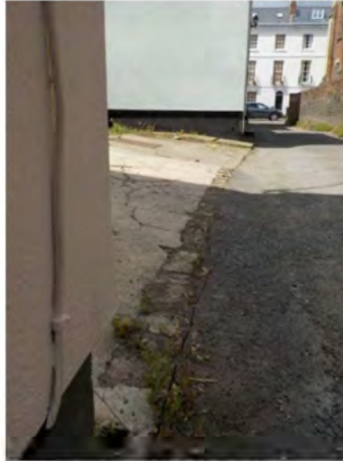
Historical remnants of fence posts, brick wall line and gate hinge [on 1 Chapel Lane]
